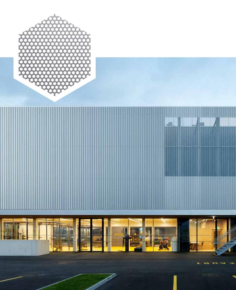
Raiffeisen Sportpark, Graz: prismatic architectural profile made of ROOFINOX CLASSIC with perforated sections
